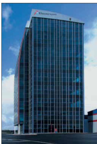
Electrium's purpose built Commercial Centre in Cannock, Staffordshire
